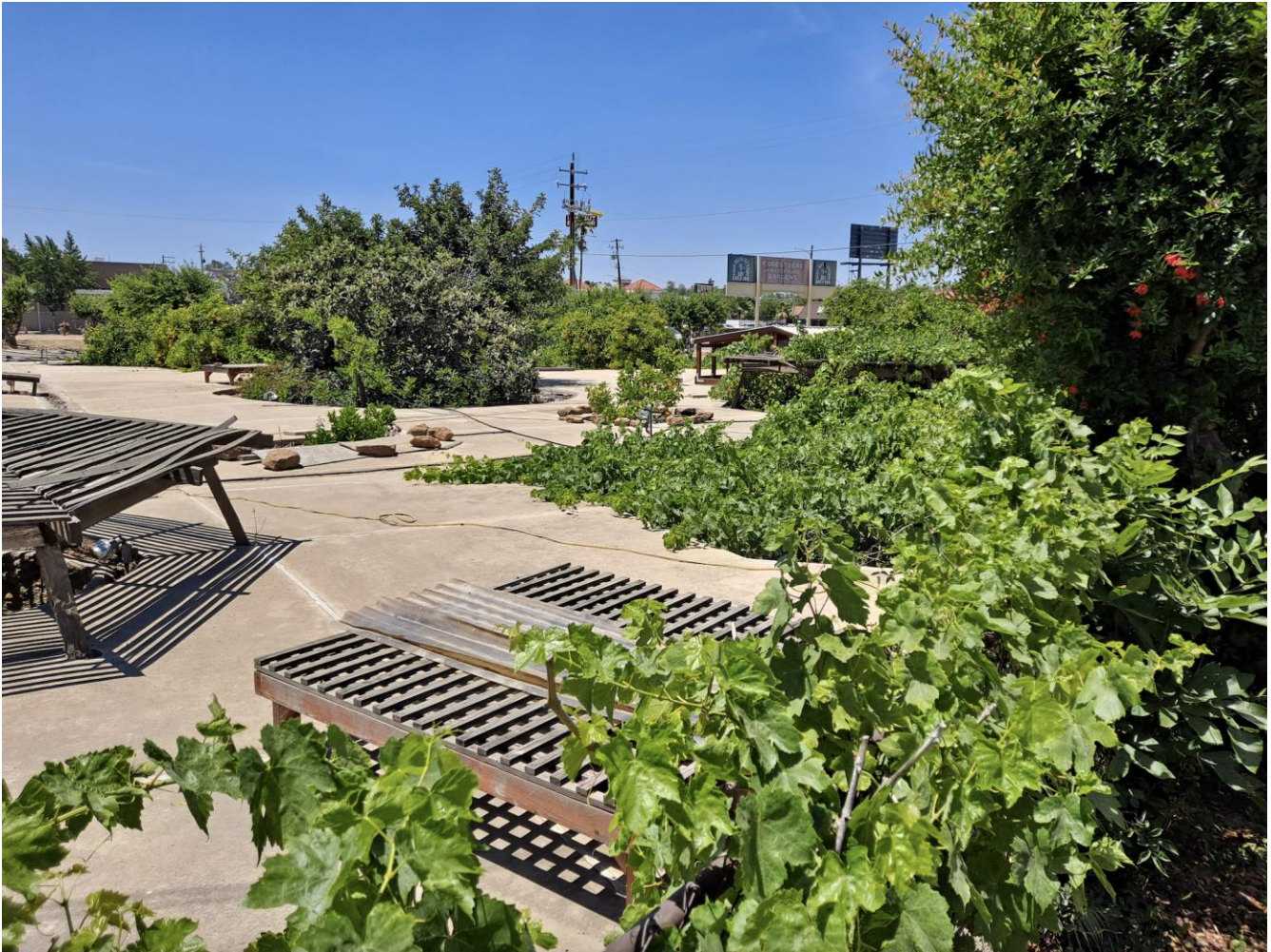
The view from above: grapevines and tree tops poke out through the skylights and courtyards below. When Forestiere wanted fruit, he simply went up to ground level, reached over, and picked the fruit.
